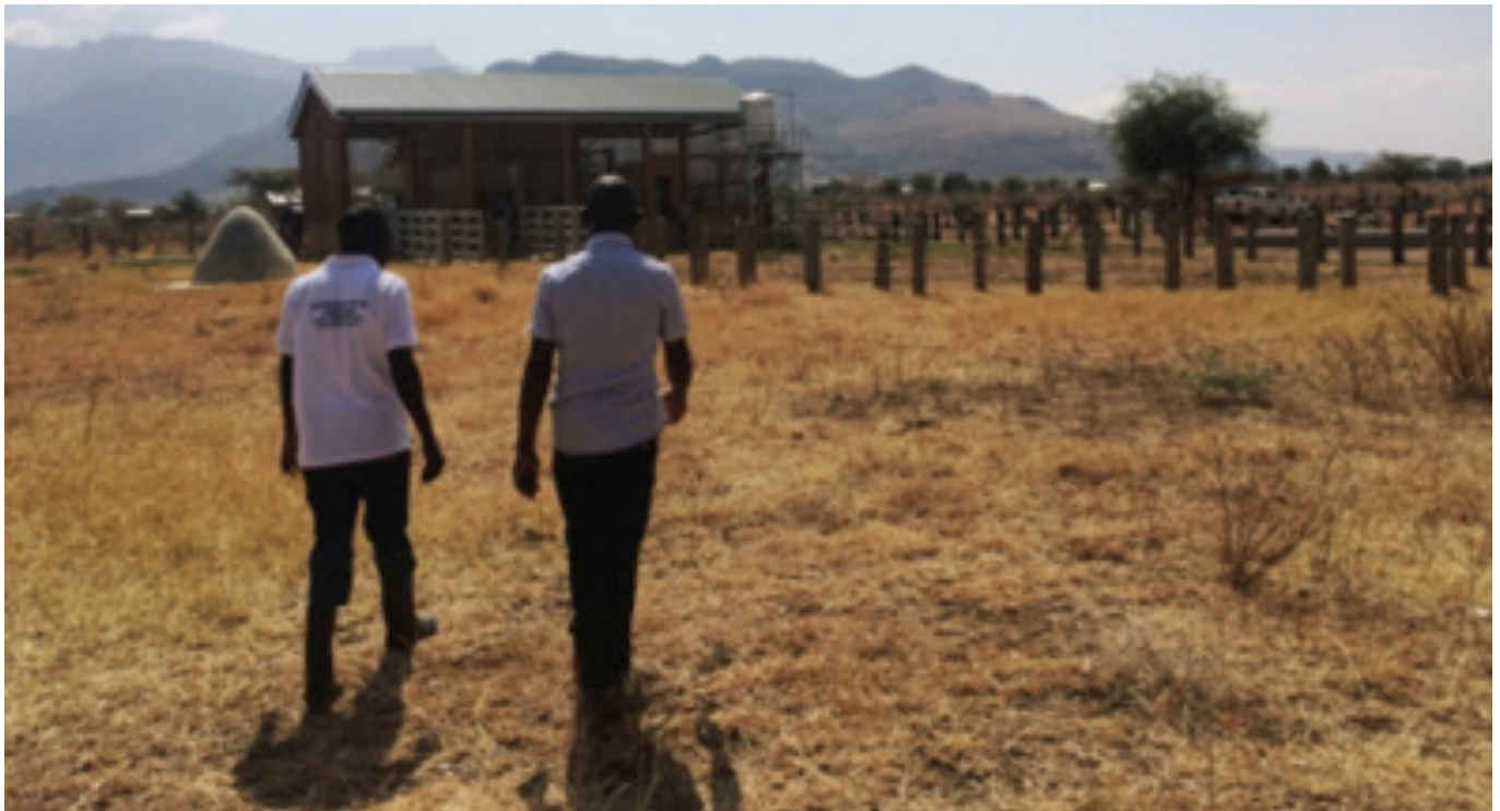
KACC Coordinator and Moroto Municipal Council Veterinary Doctor inspecting the newly constructed Slaughter house for Moroto Municipal Council during joint monitoring.
