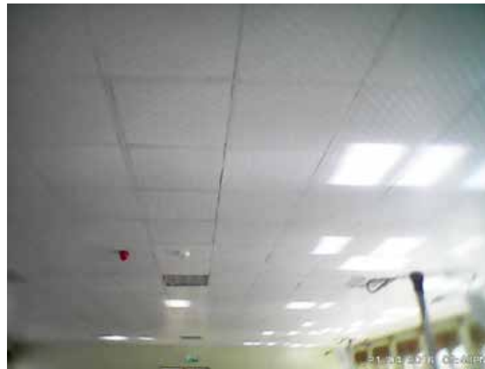
the ceiling was renovated after ACCU's intervention.
