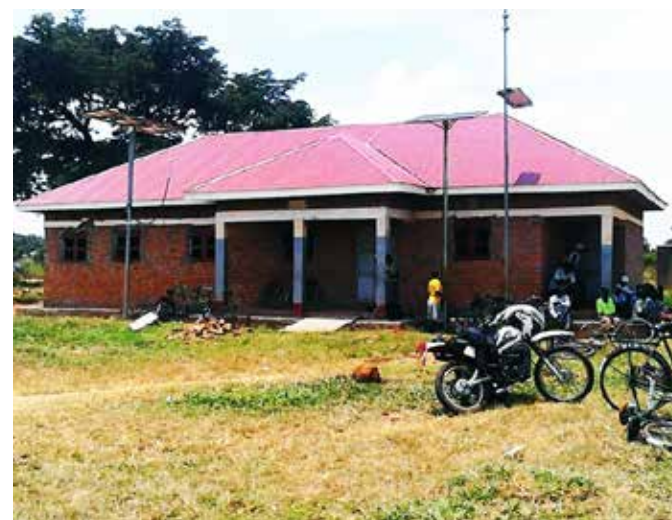
Chawente Health Centre III after rehabilitation the maternity ward. The renovation happened after ACCU engaged the duty bearers.
